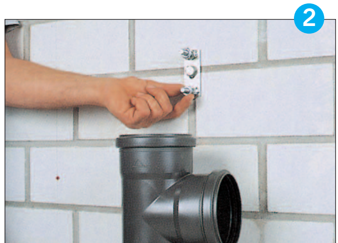
Adjusting the distance from the wall.
