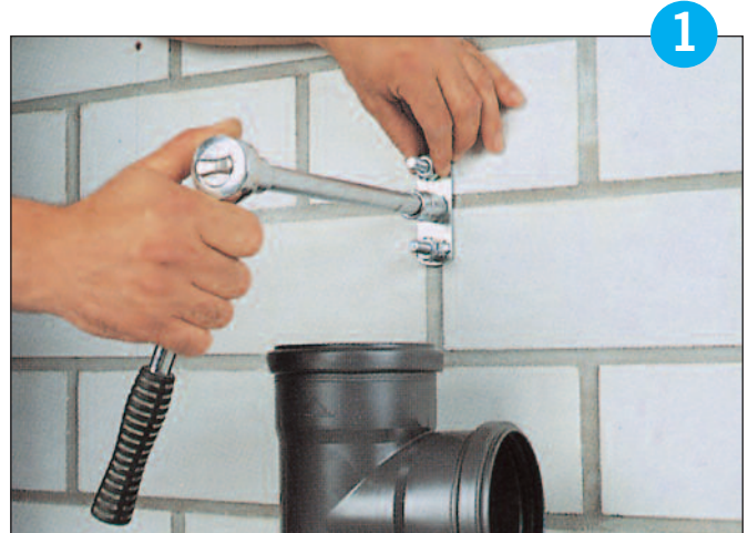
Mark, drill and fit the wall attachment.
