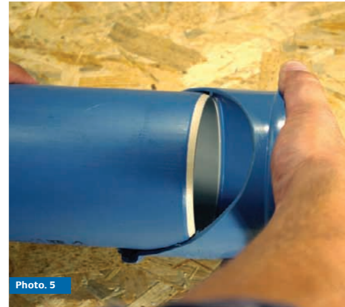
When connecting the pipe with a fitting or the socket of another pipe, push the connected pipe to the insertion depth (Photo 5) and mark a line on the edge of the socket and the connected pipe (Photo 6).
