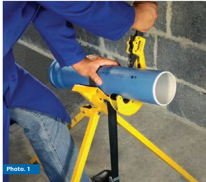
Cut the pipe using a pipe cutter (Photo 1) or a fine-toothed saw (Photo 2), with particular attention to keeping the angle 90°C.
