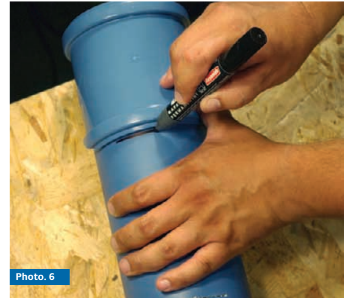
When connecting the pipe with a fitting or the socket of another pipe, push the connected pipe to the insertion depth (Photo 5) and mark a line on the edge of the socket and the connected pipe (Photo 6).
