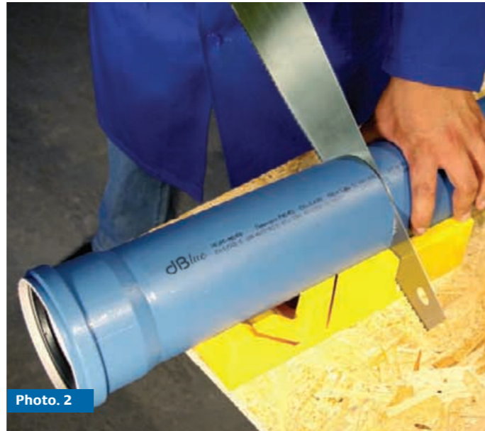
Cut the pipe using a pipe cutter (Photo 1) or a fine-toothed saw (Photo 2), with particular attention to keeping the angle 90°C.
