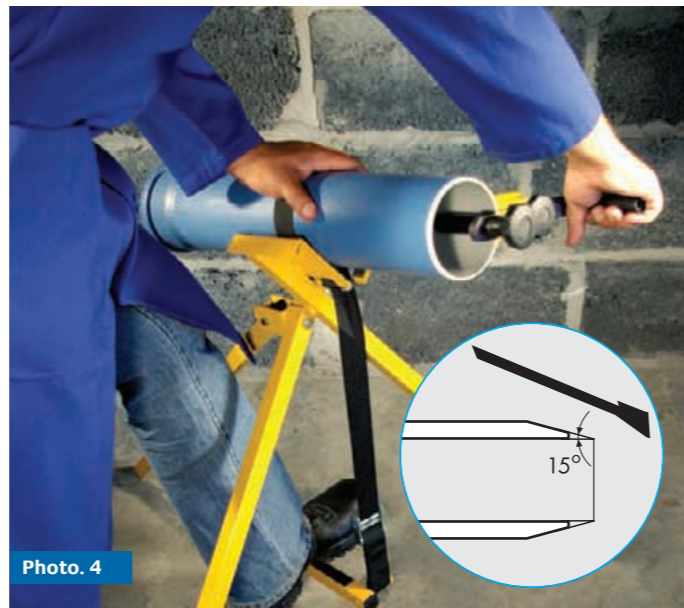
Another important factor prior to making the connections is to bevel the pipe end properly, using a chamfering tool or coarse file to provide a 15° bevel on the end of the pipe.
