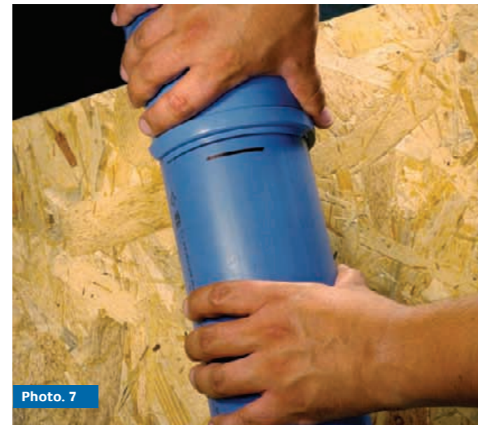
In order to allow for thermal movement, an expansion gap of between 5-10mm should be allowed within ring seal joints as each full length of pipe is installed and bracketed accordingly to ensure the gap is maintained (Photo 7).
