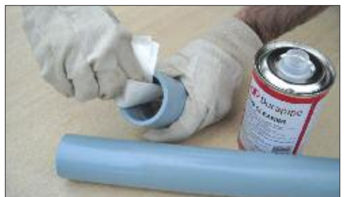
7. Clean pipe and fitting with eco cleaner.
