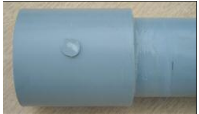
12. Using the previously marked guide, check the pipe is fully inserted into the fitting.
