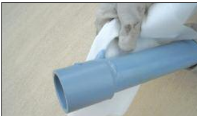
11. Cement will form a neat-bead. Wipe off excess cement with a lint-free cloth.
