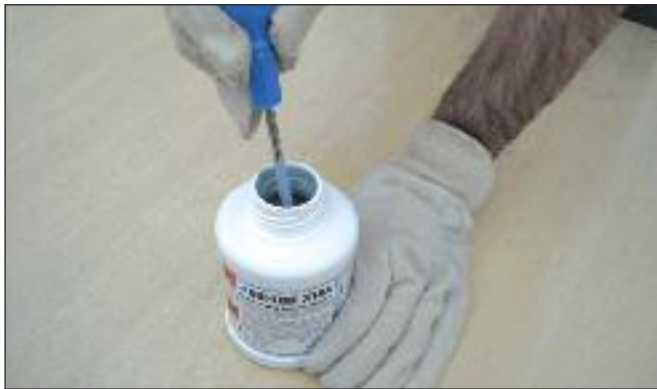
8. Stir solvent cement.
