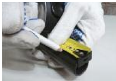
5. Mark on pipe the socket depth and a known value.
