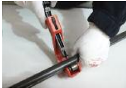
2. Cut pipe square to required length.
