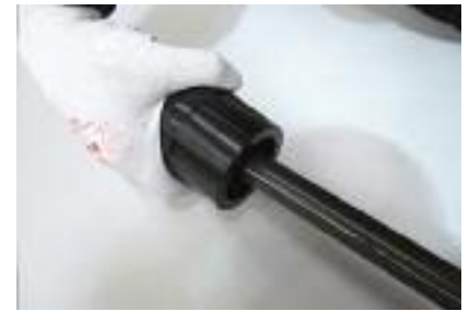
3. Chamfer and trim end of pipe.
