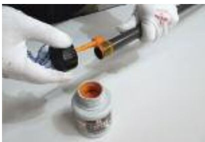
7. Apply welding polymer to fitting and pipe.
