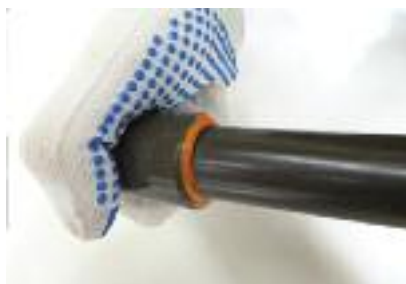
8. Push fitting straight home and hold for a few seconds.
