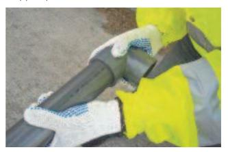
10. Wipe off excess cement from the outside of the joint.
