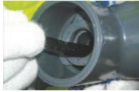
4. Without delay assemble while cement is still wet, push the pipe fully home into the fitting using sufficient force to ensure that pipe bottoms in socket. Hold together for about thirty seconds to make sure joint does not separate. With a rag, wipe off excess cement. Avoid disturbing the joint.
