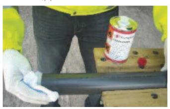
3. Using a clean brush, apply Durapipe PVC One-step cement to the carrier pipe and inner fitting. HCR-36 cement and cleaner should be used for aggressive chemicals, for more information please see page 18.
